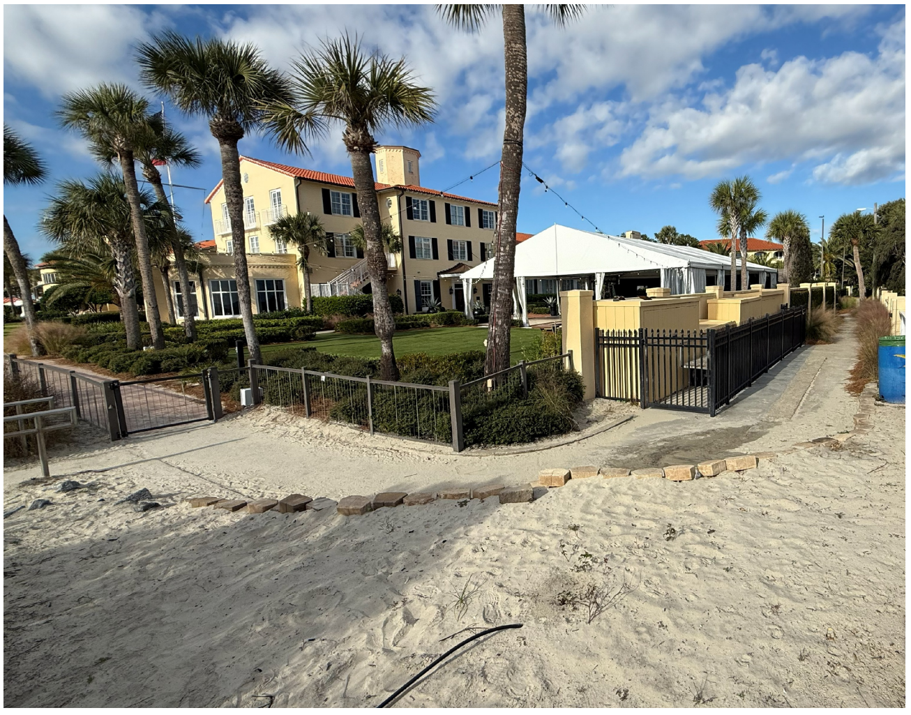
7 VIEW OF AREA LEADING TO THE EXISTING NORTHERN CROSSOVER
