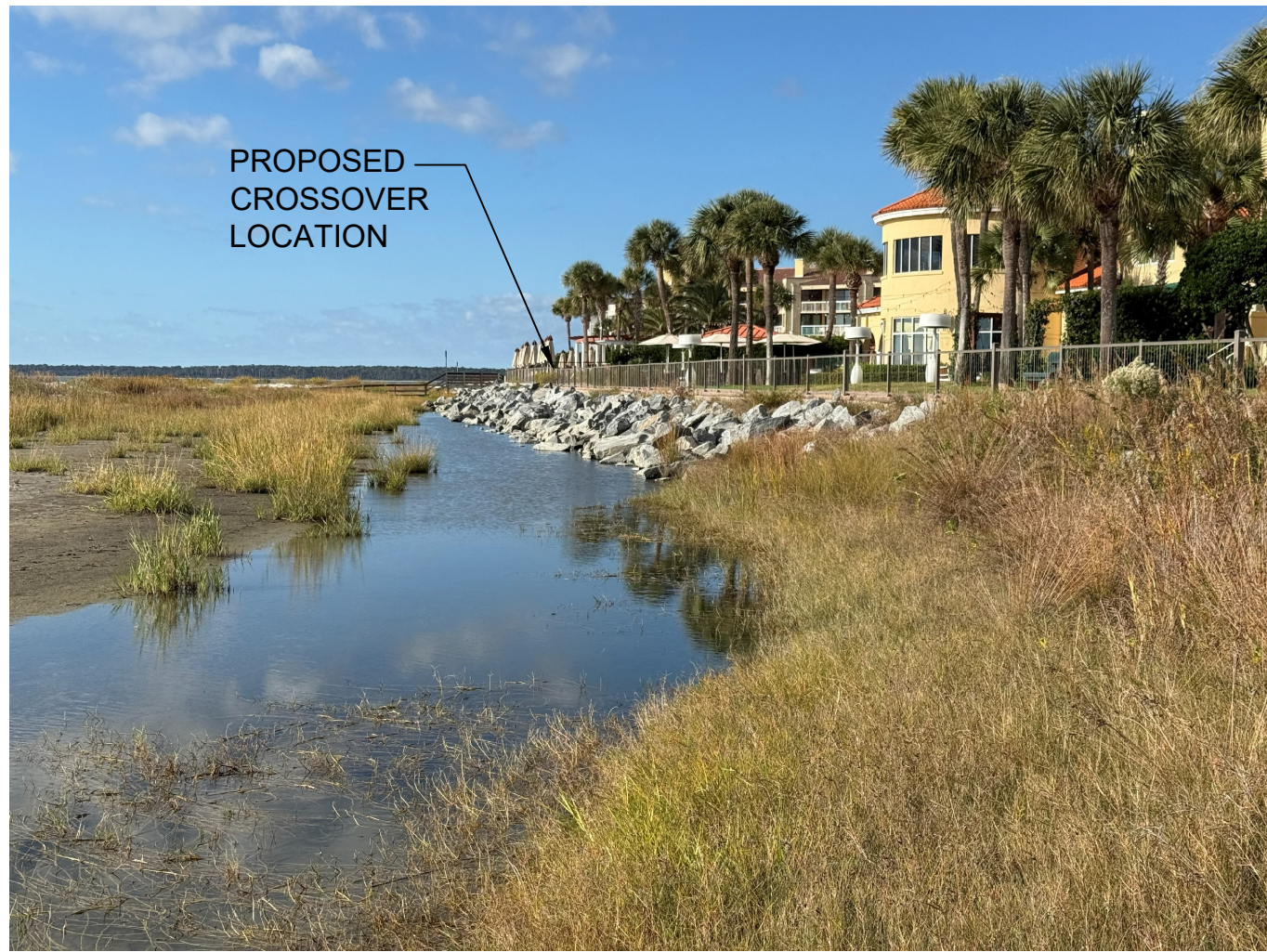
5 VIEW OF WATER IMPOUND AREA ALONG THE BEACH FRONT OF THE HOTEL
