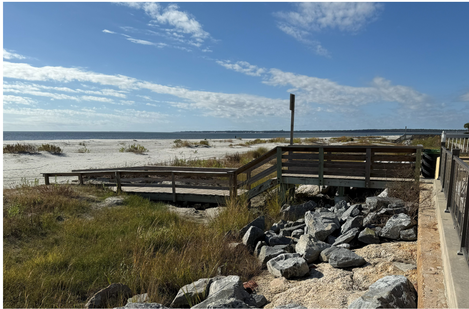
4 VIEW OF EXISTING SOUTHERN CROSSOVER POPOSED CROSSOVER TO BE SIMILAR CONSTRUCTION
